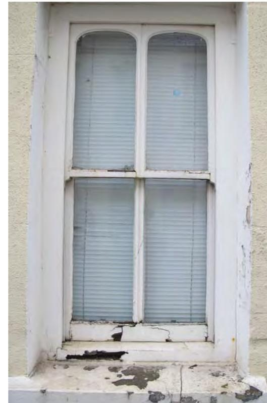
Example of decay to Timber Sash Window through poor maintenance
