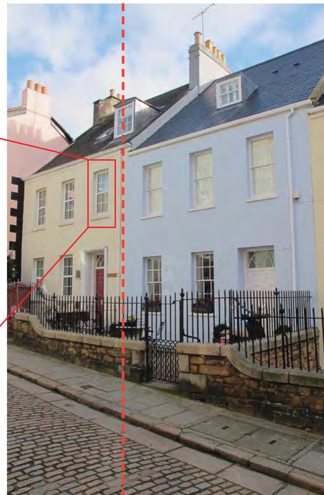
Example historic window replaced with inappropriate UPVC units      Example historic glass detail retained
