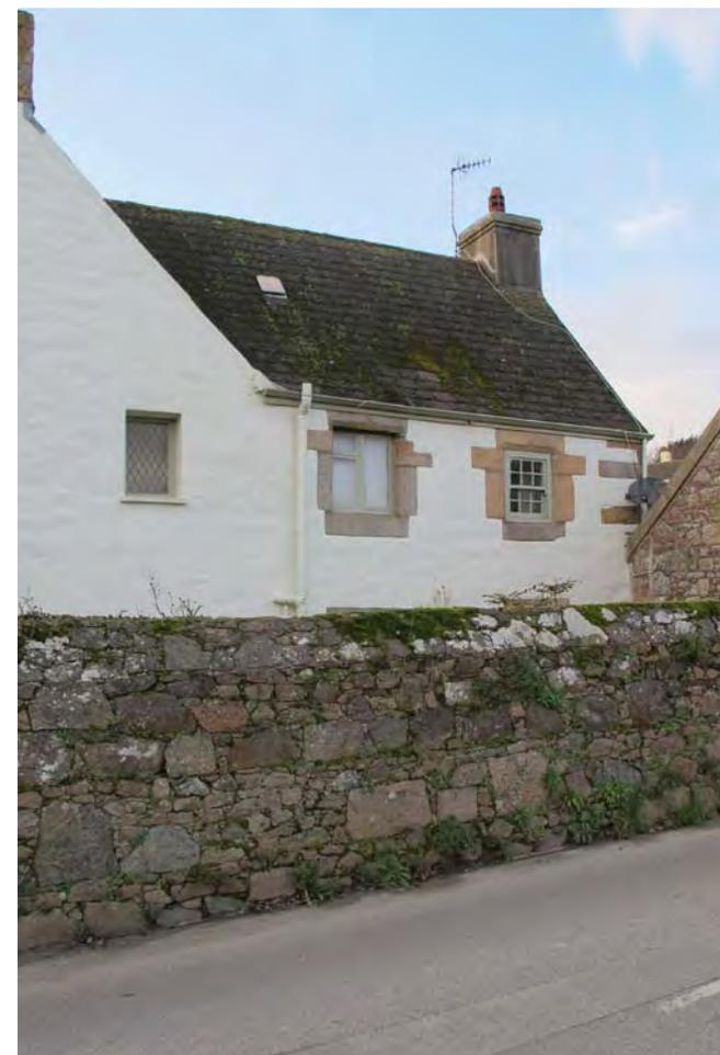
Example timber frame fixed leaded light, casement and vertical sliding sash
